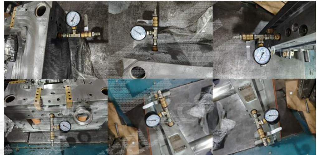
Pressure Test After Replacing Water Transport Components
